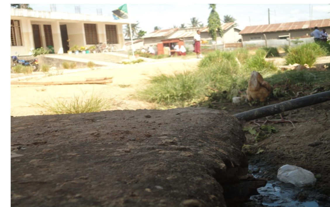
Waste water (sewage) from the residential area to the school compounds.
